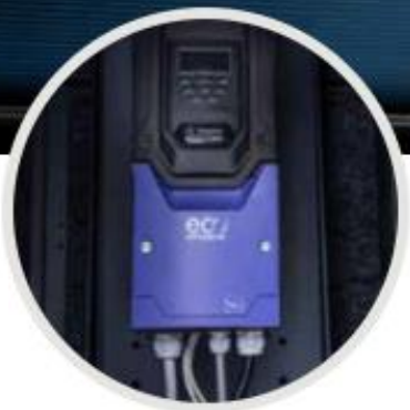
Variable Speed Drive
